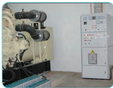
Upgrading Hospital Melaka's Genset capacity
